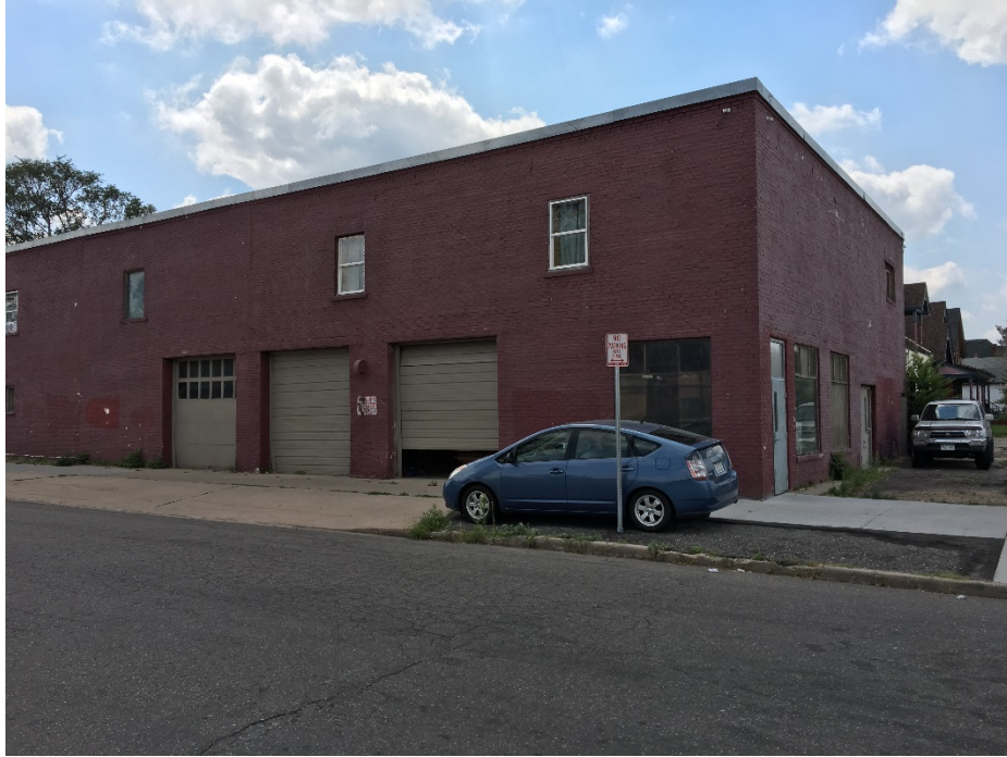
This industrial building is located south of the subject site, across 37 th Ave.
