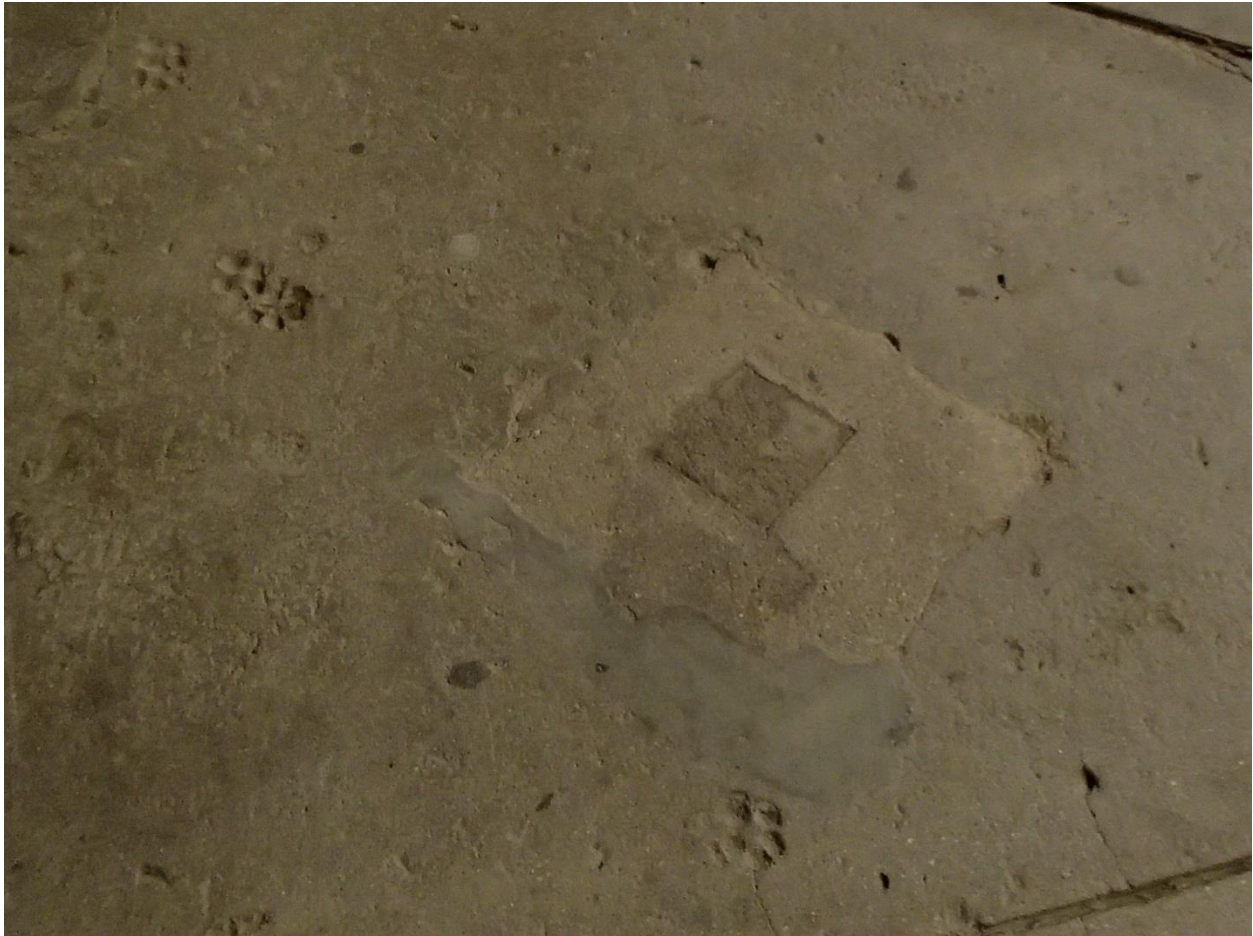
Figure 24. Infilled square post hole and dog footprints at the location of the auction arena, walled off from the main arena from 1953 until the early 1960s. Photographed February 9, 2016, Kathleen Corbett.
