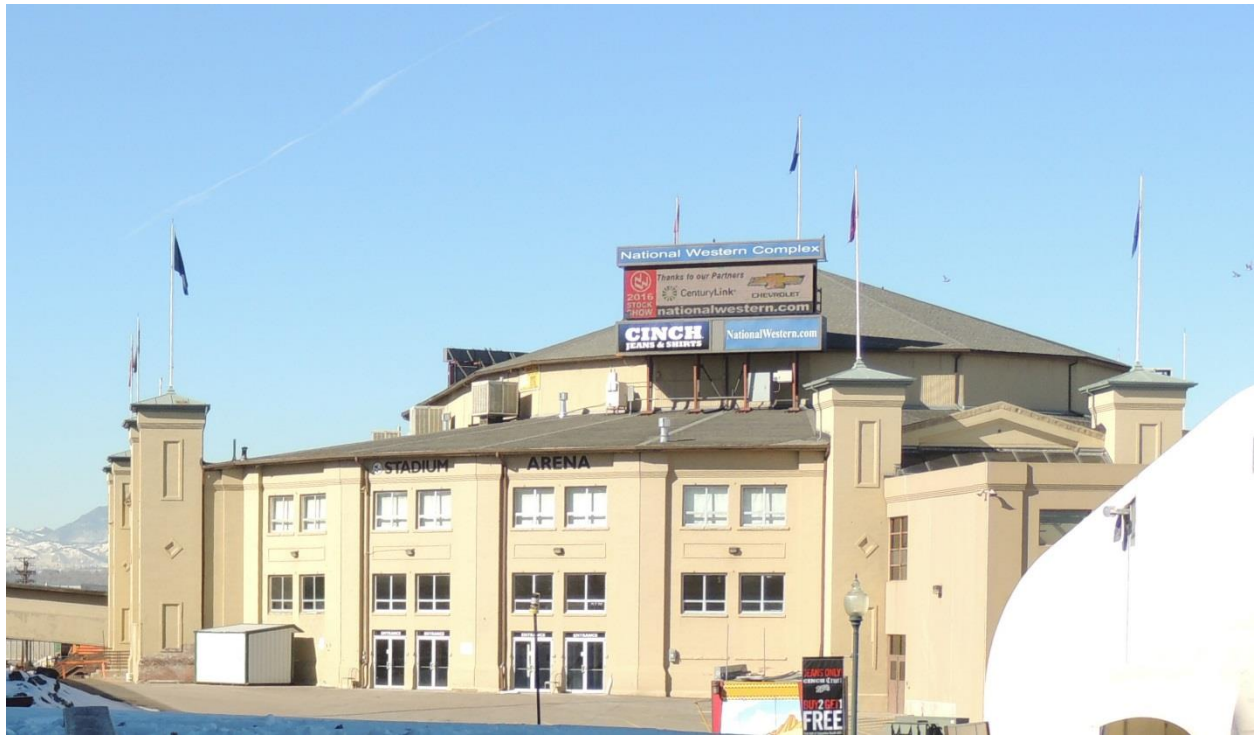
Figure 5. The Stadium Arena, showing the roof configuration of upper monitor roof centered over an oval hipped roof. Facing west. Photographed February 9, 2016, Dianna Litvak.
