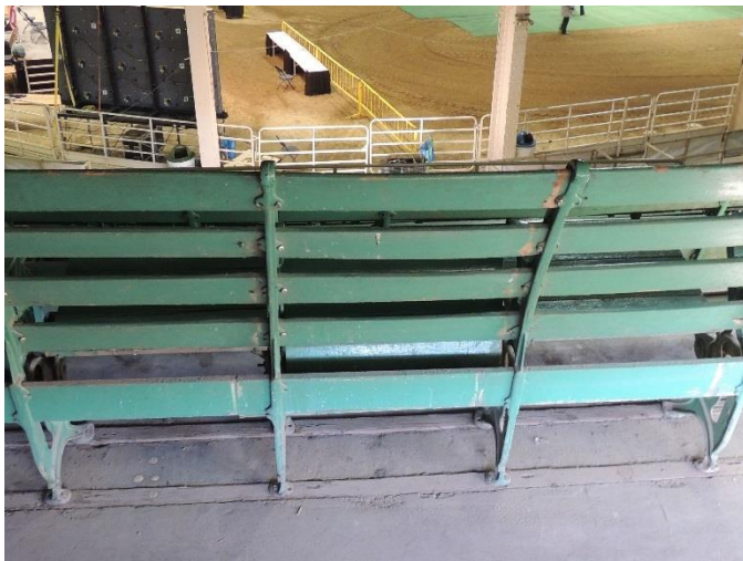
Figure 19. Stadium seating showing wooden slats embedded in the concrete risers. Photographed January 21, 2016, Dianna Litvak.
