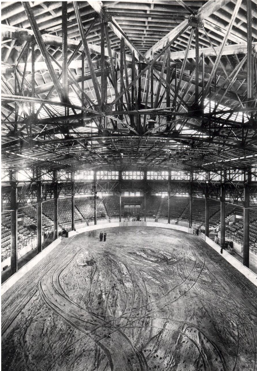
Figure 13. Historic photograph of the nearly completed National Amphitheater, showing the structural system of the roof and the configuration of the support beams. Courtesy NWC archives, February 9, 2016.
