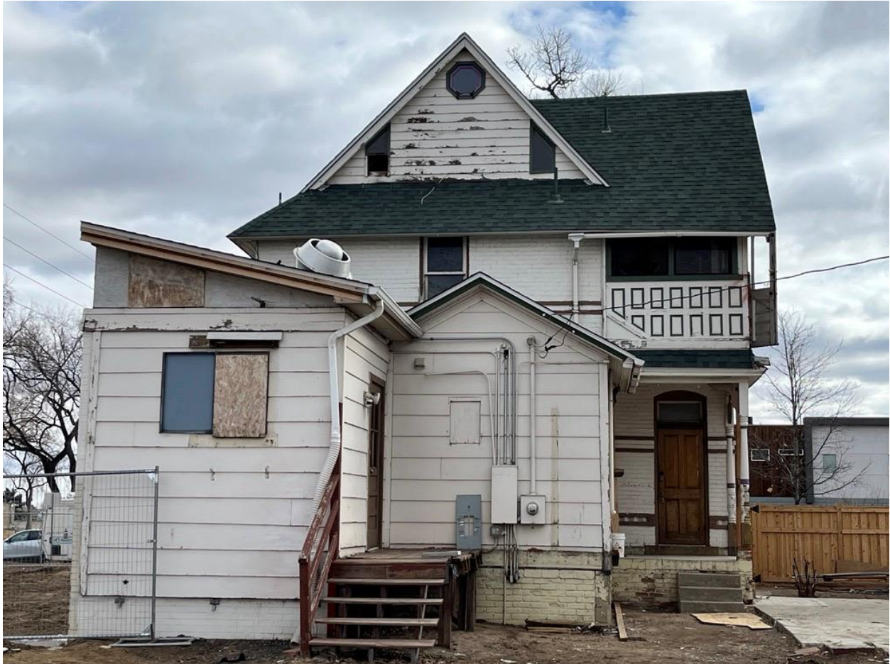
3435 Albion Street, rear facade, with additions
