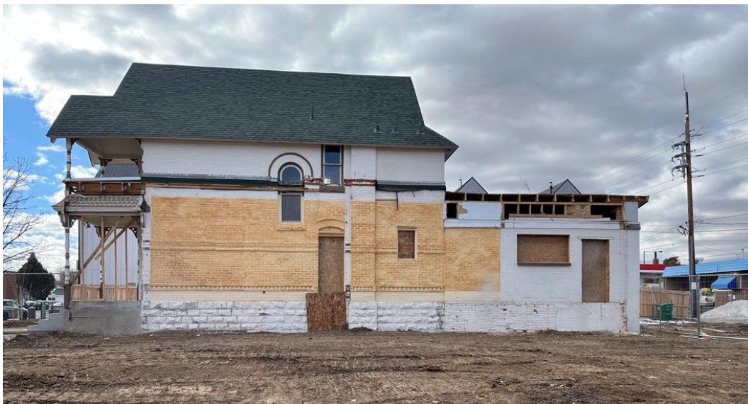
3435 Albion Street, side façade and rear additions
