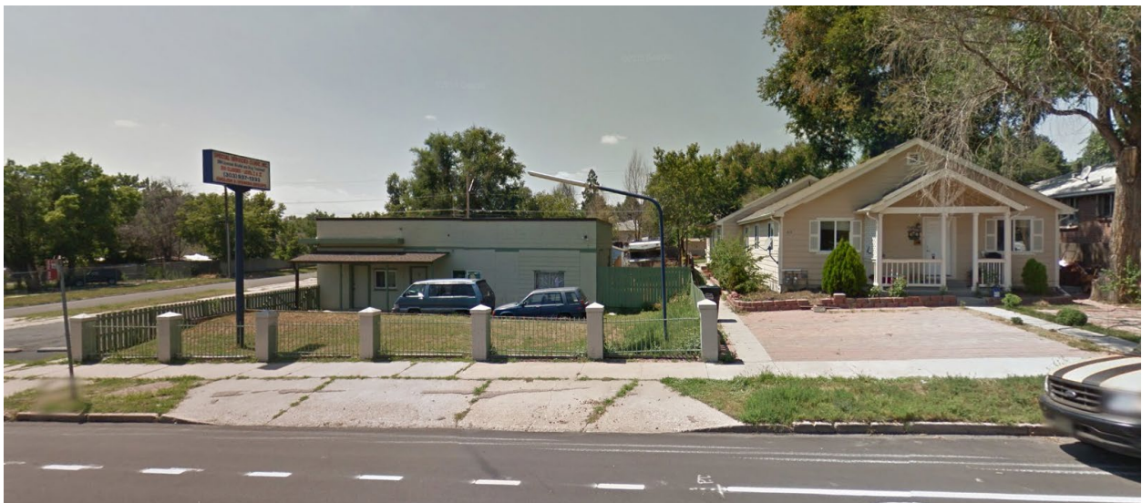
Surrounding Properties Looking West
