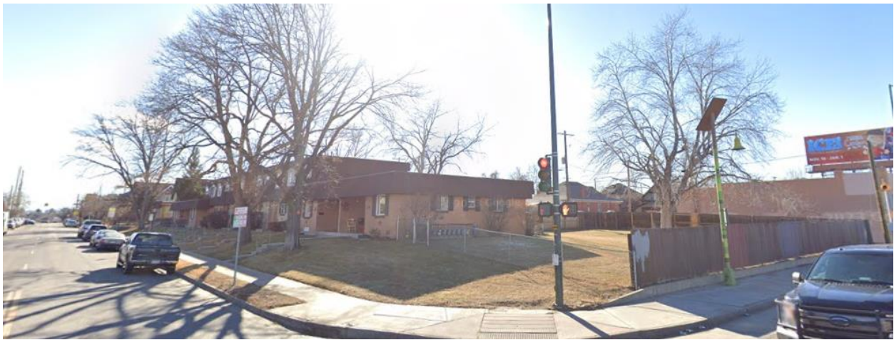
Site – View of the subject property looking southwest from Colfax Avenue and Knox Ct. (Source: Google Maps)
