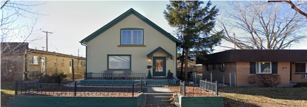
South – looking west from Knox Ct. (Source: Google Maps)
