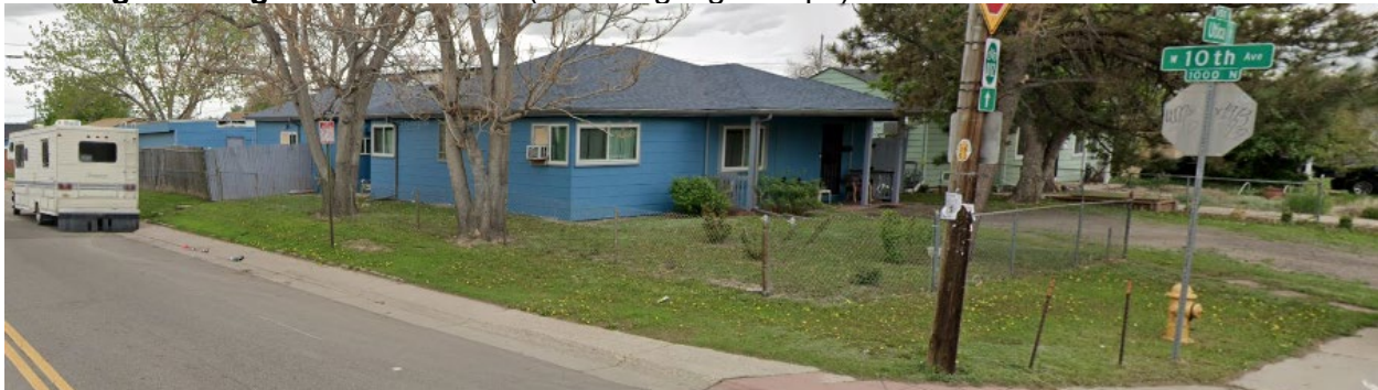
Subject property – Looking southeast from the corner of West 10 th Avenue and North Utica Street
