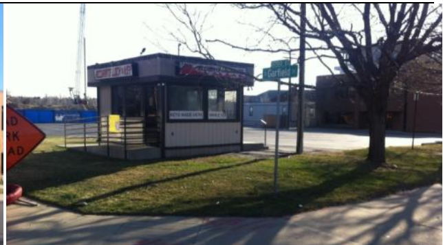
View looking southwest from Garfield and Alameda
