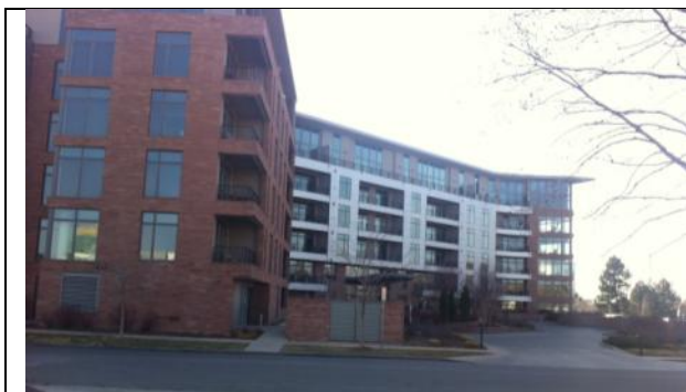
View from site looking west across Monroe Street
