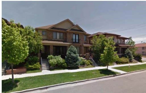
East - facing the subject property along Jackson St.
