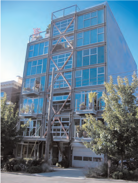
Update the zoning along West Colfax Ave. to encourage multi-storied, mixed-use development along the transit-rich corridor.
