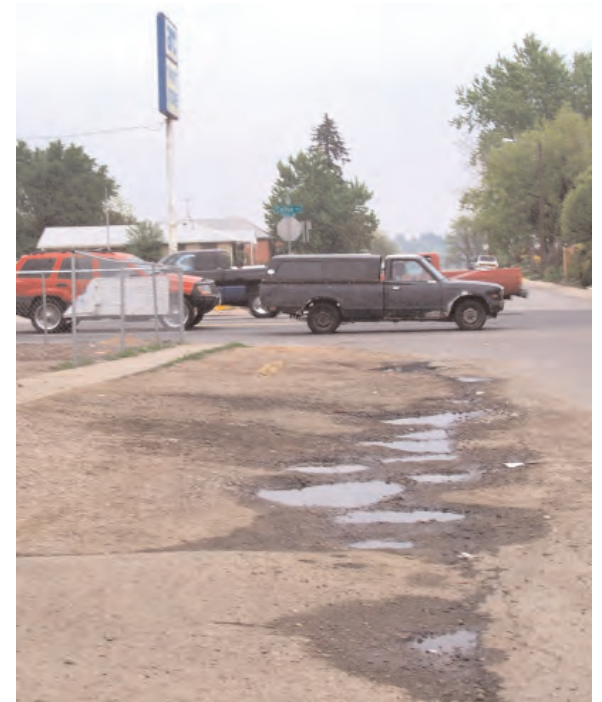
Asphalt covered tree lawns, a lack of curb and gutter and unpaved alleys are signs of aged and neglected infrastructure.
