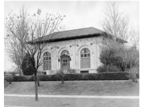
Dickenson Branch Library building at Conejos and Hooker Streets.
