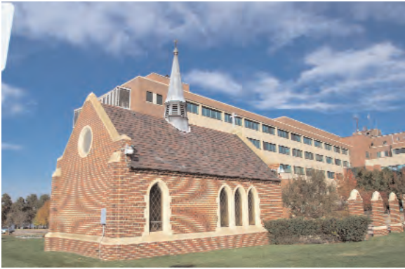
The Saint Anthony's Hospital Redevelopment Task Force recognized the existing chapel as an important reference to the site's history and recommended that future redevelopment incorporate it as a focal point of the town center.
