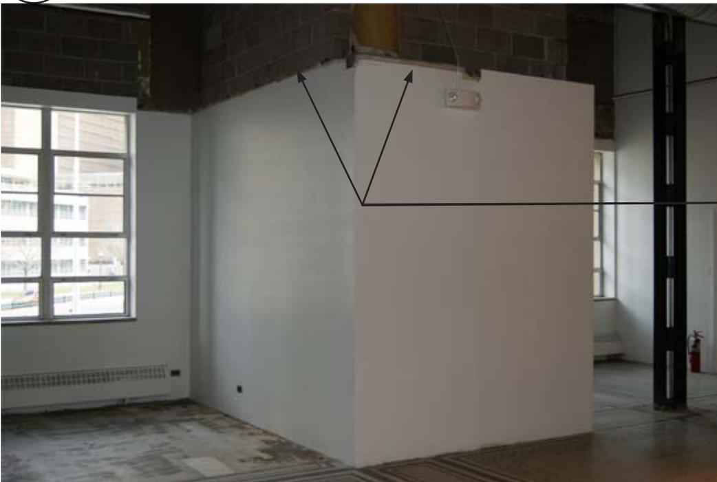
Complete/finish termination of (E) plaster and/or gyp board wall around elevator (including east side.) Paint white to match adjacent wall
