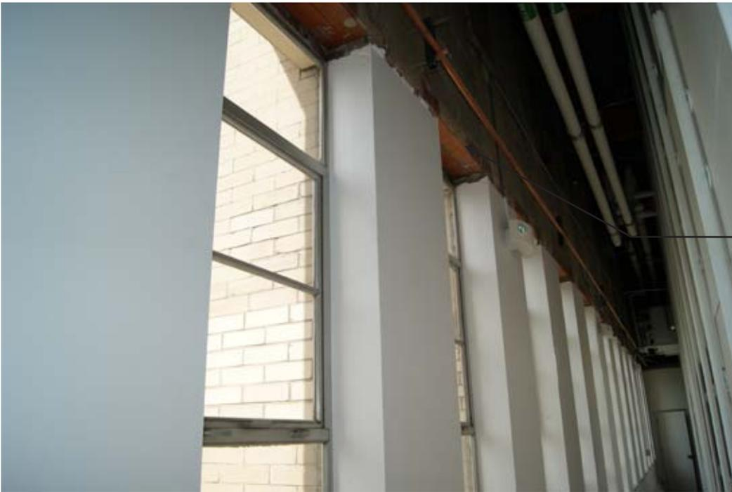
Provide continuous 1'D x 2'H furred wall w/2-1/2" metal studs & 5/8" gyp board abv (E) window head. Extend gyp bd into existing opening at head to conceal (E) lintels
