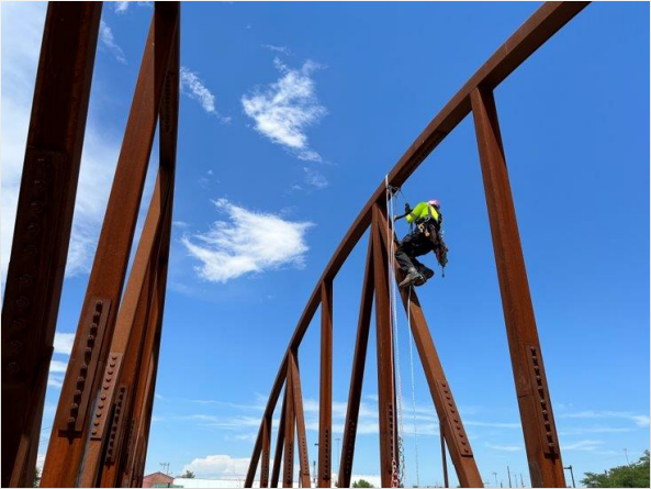
2024 Bridge Inspection Program
