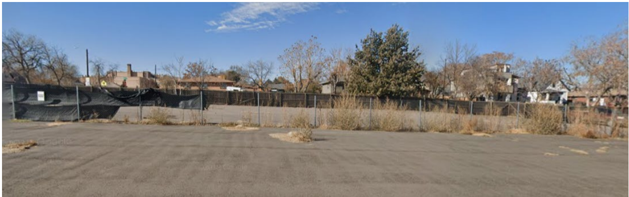
Site – from alley (Source: Google Maps)
