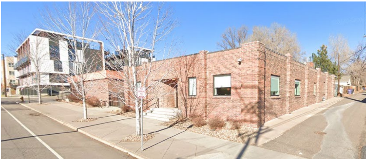
West – property directly west of the subject property looking northwest from West 29 th Avenue
