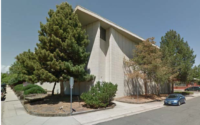
Northwest corner of Conejos Place and Stuart Street, viewing existing sanctuary on the subject site.
