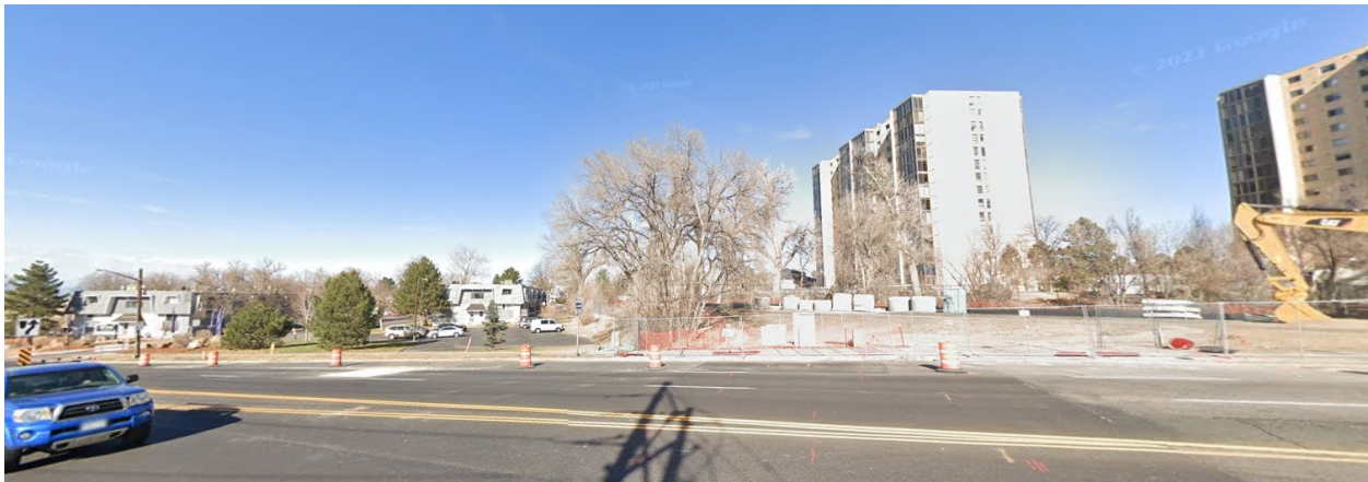
North - Looking north from S. Parker Road
