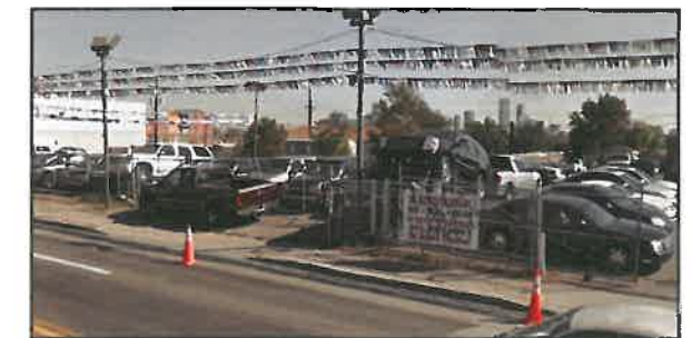
EAST SIDE (STA 31+88)
