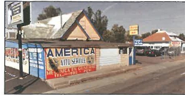
WEST SIDE (STA 38+35)
