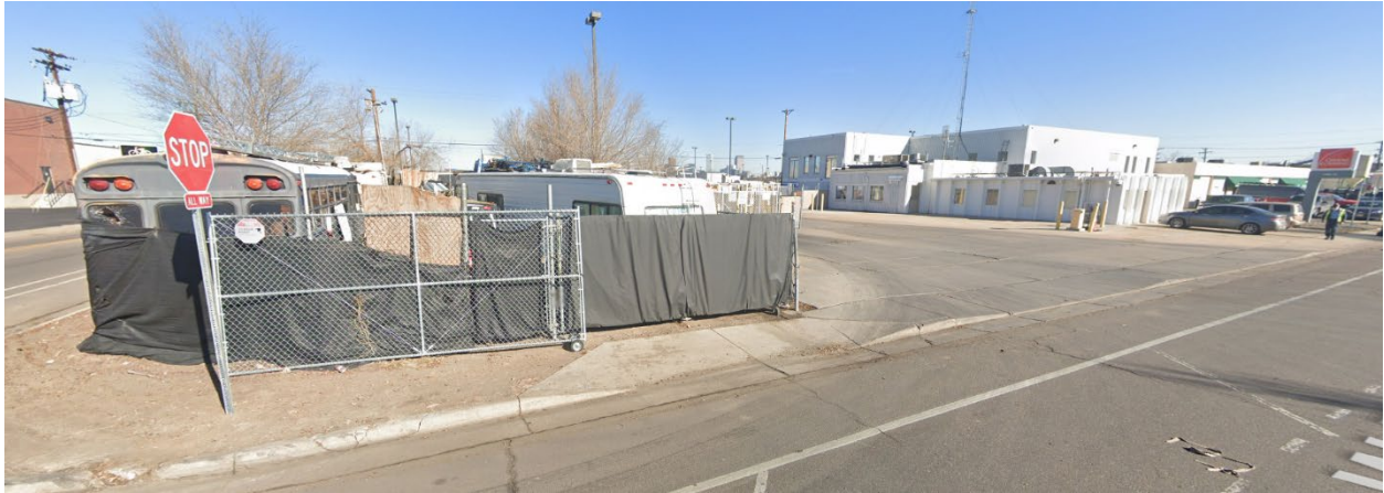
North - Looking northeast from W. Bayaud Avenue
