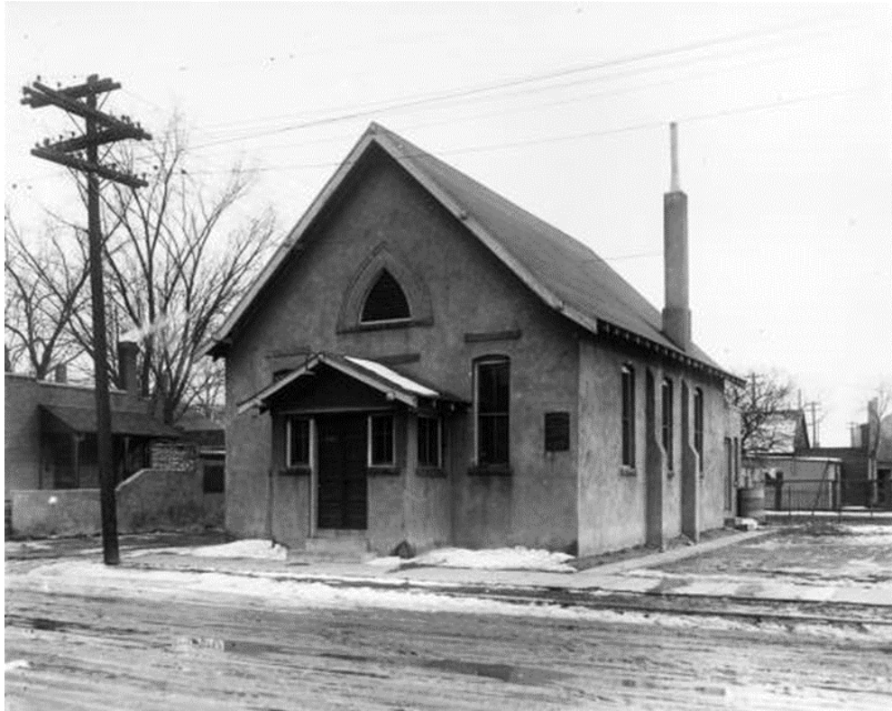
Historic photo of front, north façade Circa 1930
