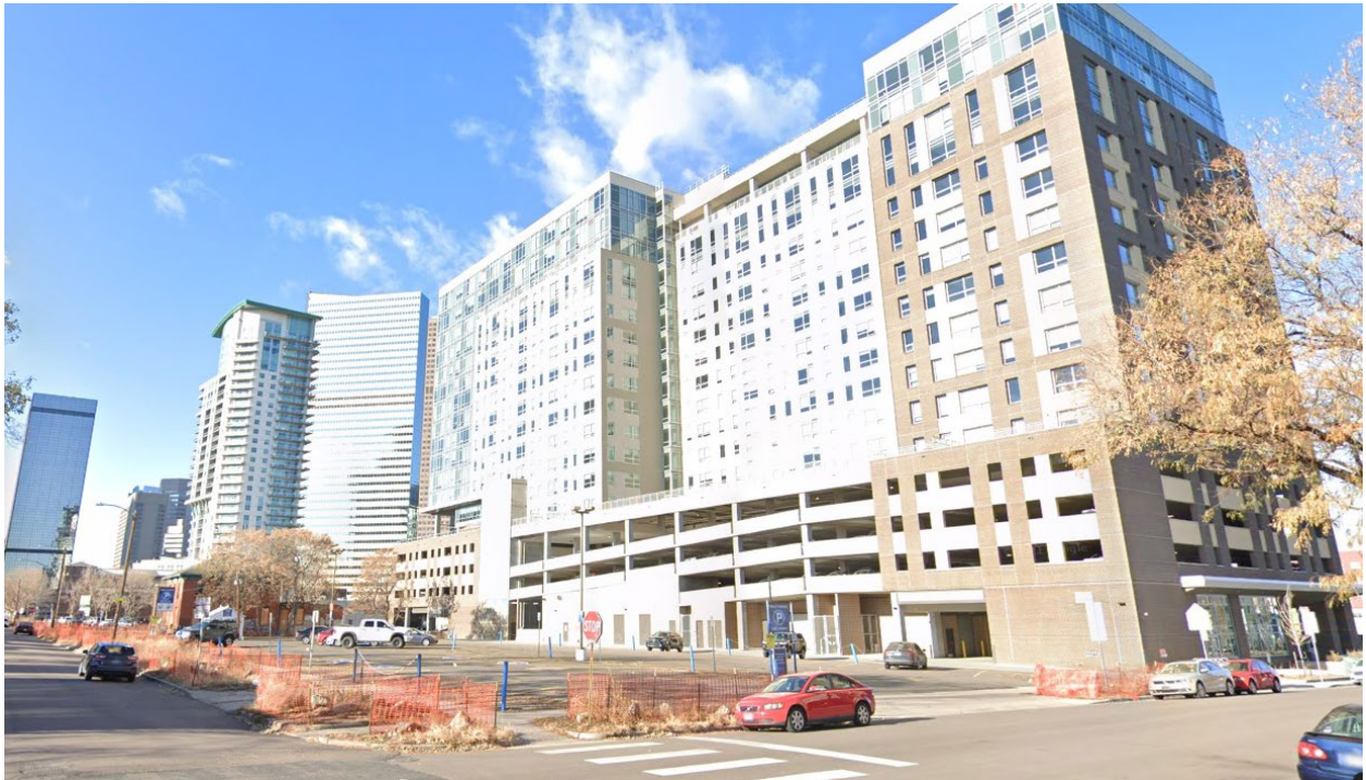
Site: Looking southwest from Glenarm Place.
