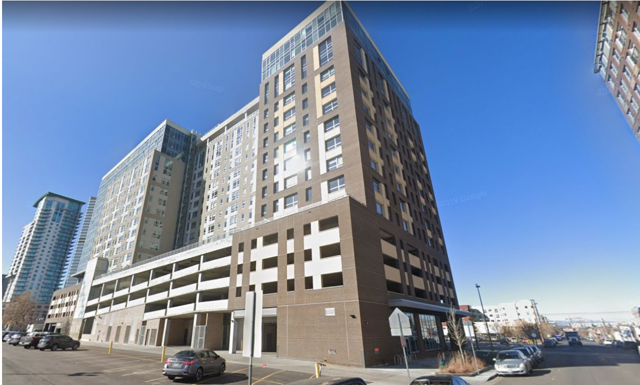
Northwest of site: Looking southeast from 22 nd Street.
