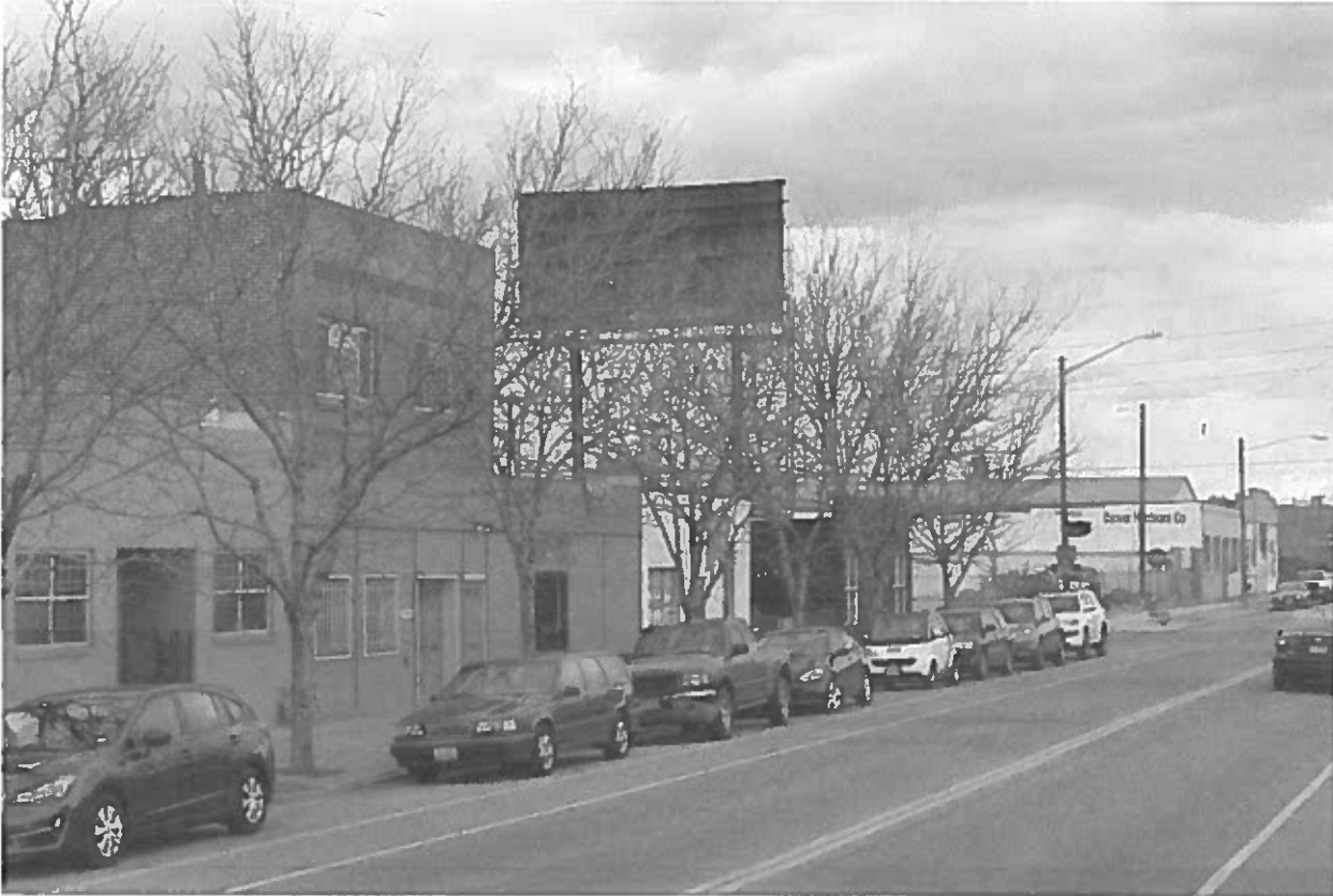
Close up looking north on Larimer at Denver Hardware site
