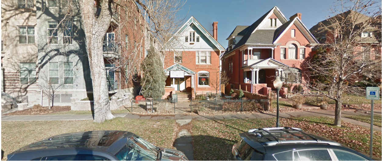
Subject property, looking north on East 17th Avenue.
