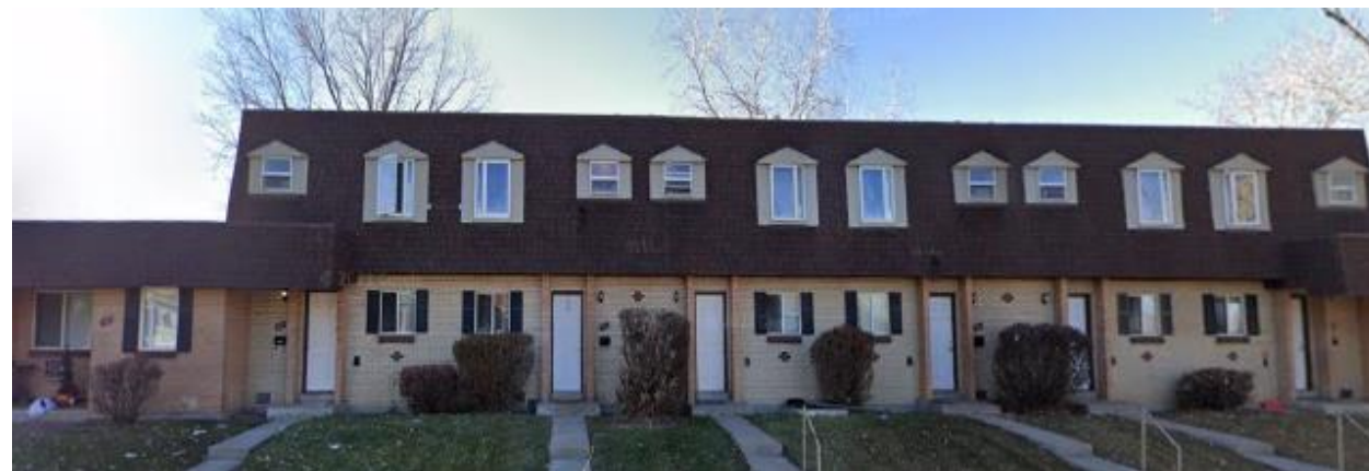
Subject Property looking west
