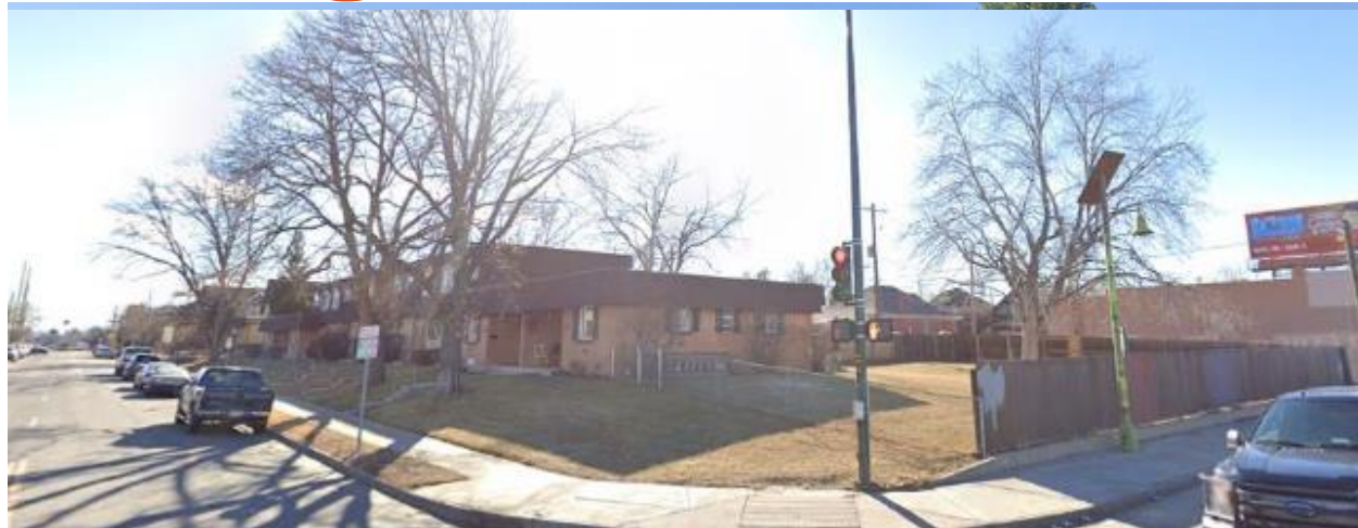
Subject property looking southwest
