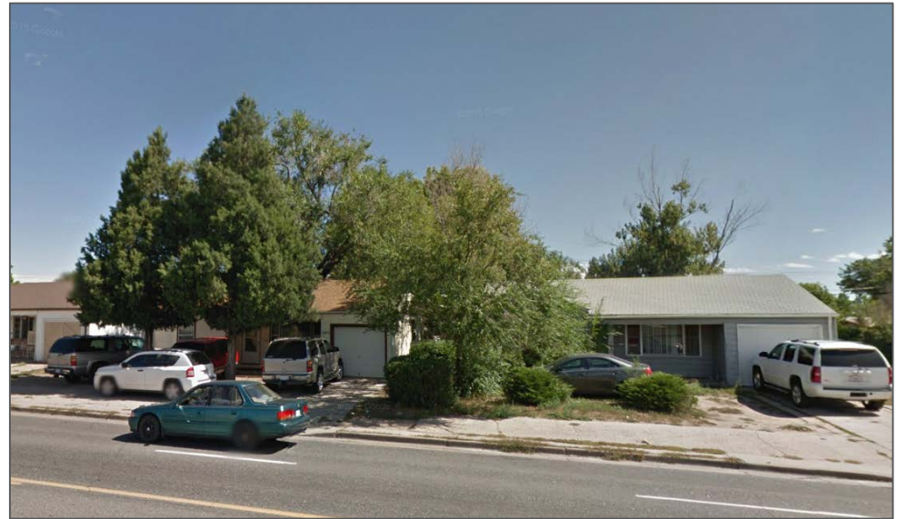
Existing attached sidewalk through south segment of project poses safety issues due to proximity to high volume roadway
