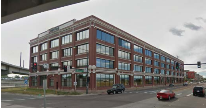
Four-story office to the east of the subject site on S. Broadway
