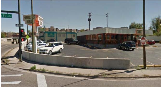
One-story restaurant to the south of the site on S. Santa Fe Dr. and W. Mississippi Ave.
