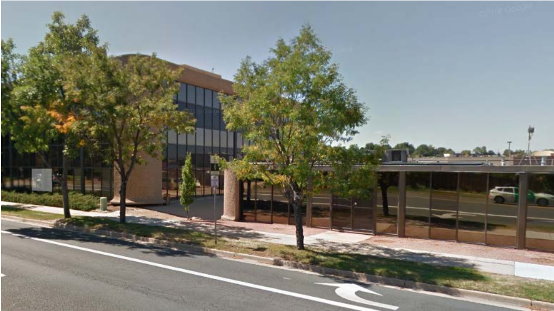
Subject Site, looking west
