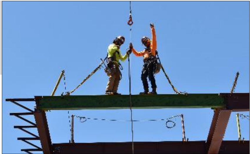
Denver Botanic Gardens: Freyer – Newman Center Topping Off
