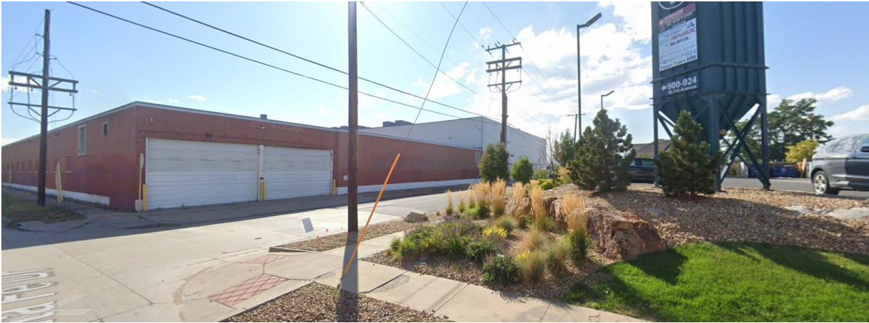
View of the subject property at 50 S. Kalamath St. from S. Santa Fe Dr. and W. Ellsworth Ave., looking southwest.
