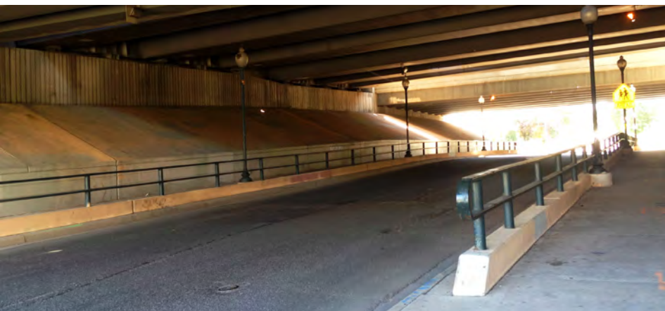
The Lincoln Street Underpass is dark.
