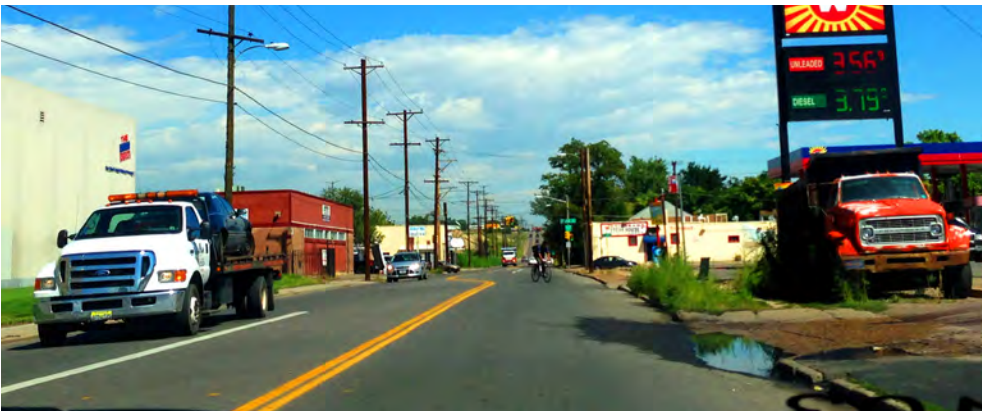
The middle section of Washington Street is narrow, and the facilities that are provided vary from one block to the next. The block shown here between 50th and 51st Avenues features two travel lanes, a turn lane, and attached sidewalks. Many businesses are located close to the right of way.
