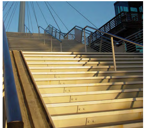
The Millennium Bridge in the Central Platte Valley features a wheel well for cyclist ease. A similar approach could be used to formalize the social path at the corner of 44th Avenue and Broadway.
