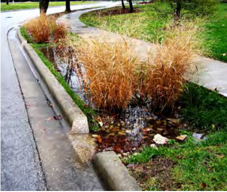
Green Infrastructure improves water quality by filtering pollutants out of stormwater before it travels off-site.
