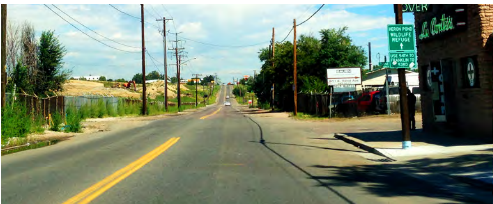
The Northern section of Washington Street is narrow and will need to be designed to effectively transition to the future Adams County cross-section.
