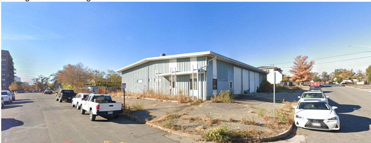
View of 4155 North Jason Street, looking southwest.
