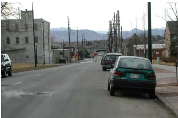
Inconsistent sidewalks are found throughout the industrial area of the neighborhood.
