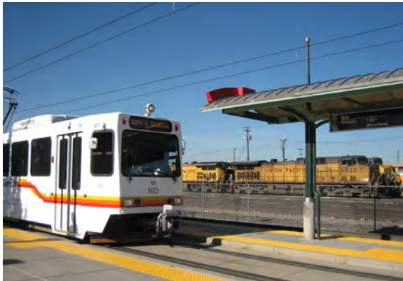
The 10th and Osage light rail station provides convenient access via the Central Corridor
