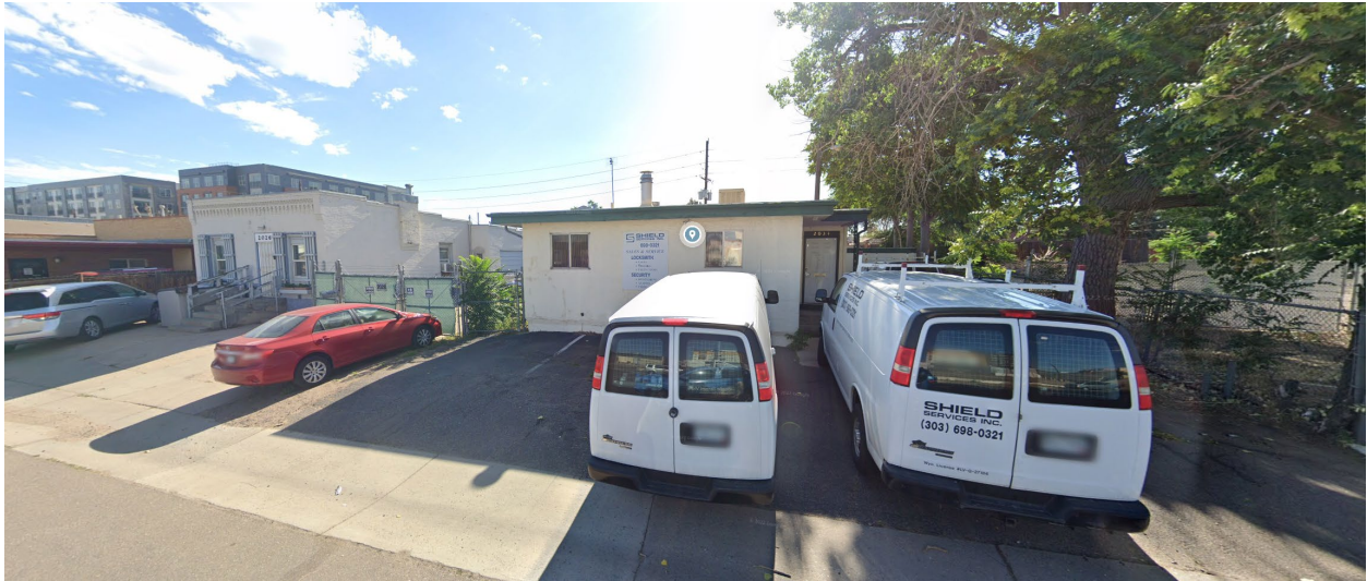
North – from South Bannock Street looking northeast
