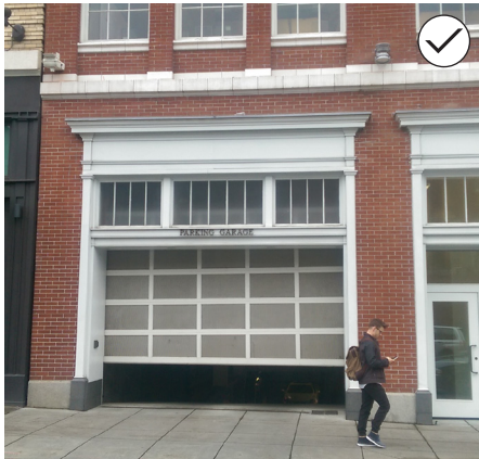
Limiting the width of vehicle access points can help minimize impacts on pedestrians.
