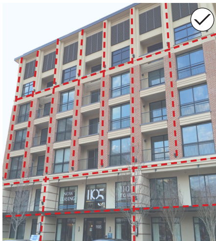
15. Where balconies and terraces are provided, they should be integrated into vertical and horizontal articulation systems.
