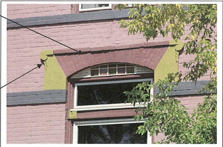
5. South Window Detail
