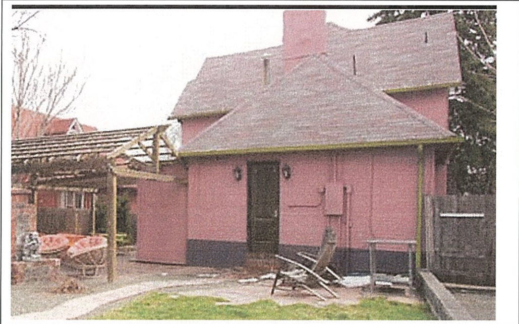
10. View of North Elevation
