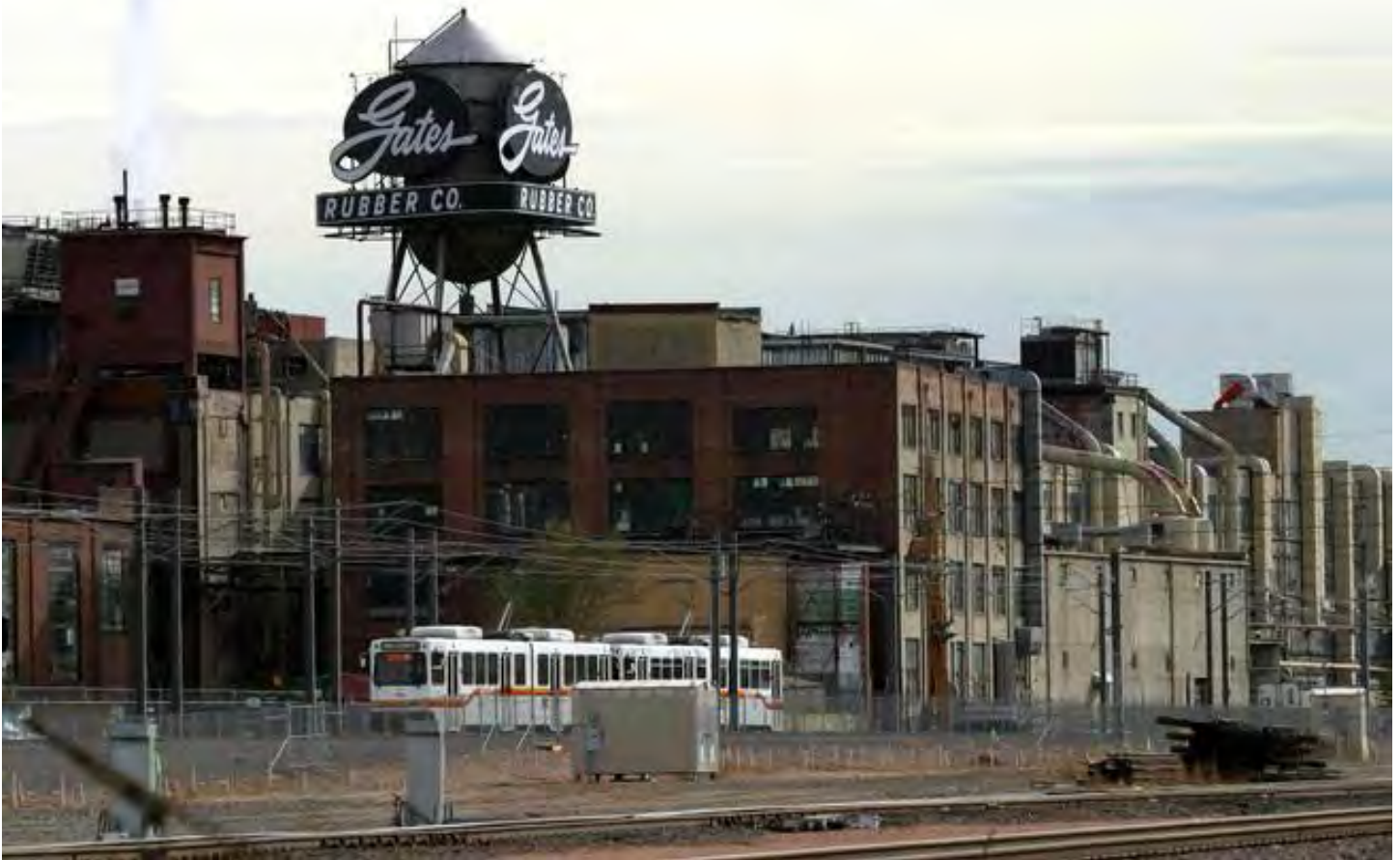
Gates Rubber Factory prior to demolition
