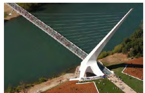
Signature pedestrian and bicycle bridge.
