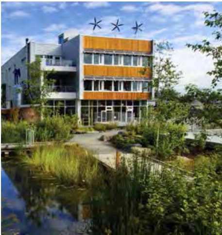
Example of ground floor residential units set-back from Santa-Fe corridor. Setback may incorporate water quality features.
