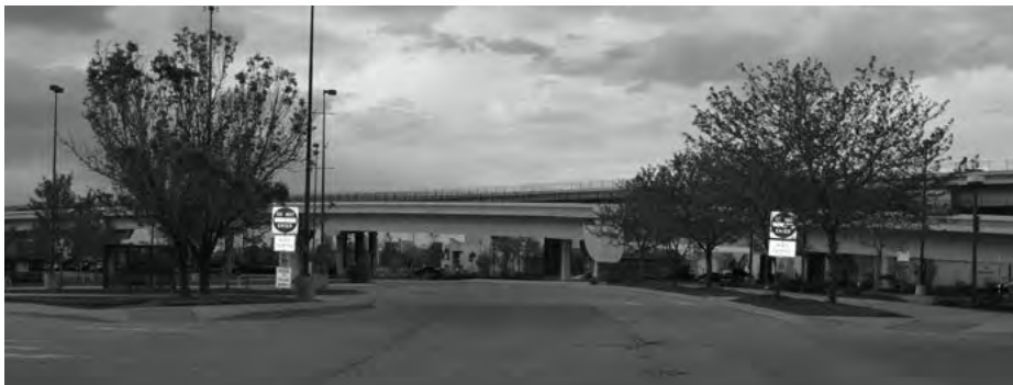
Existing I-25 and Broadway Station parking lot
