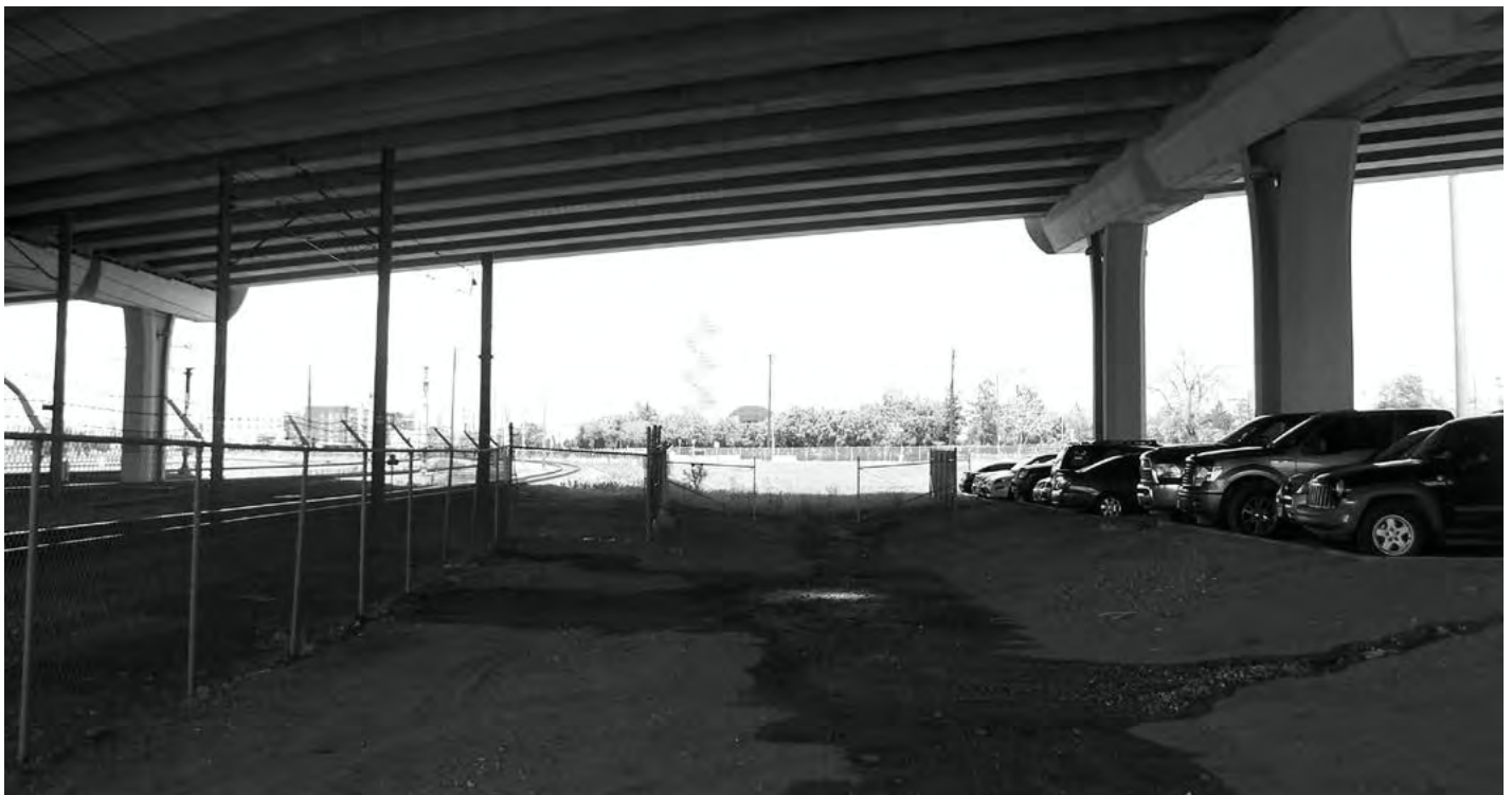
Existing conditions under the I-25 overpass.
