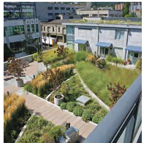
Green roof as usable outdoor space helps to reduce the heat island effect
