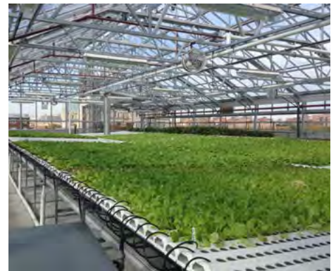
Rooftop greenhouse. Bronx, NY
