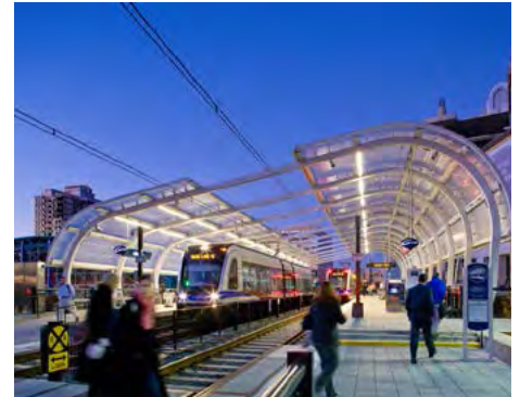
Unique station canopy as a placemaking element.
