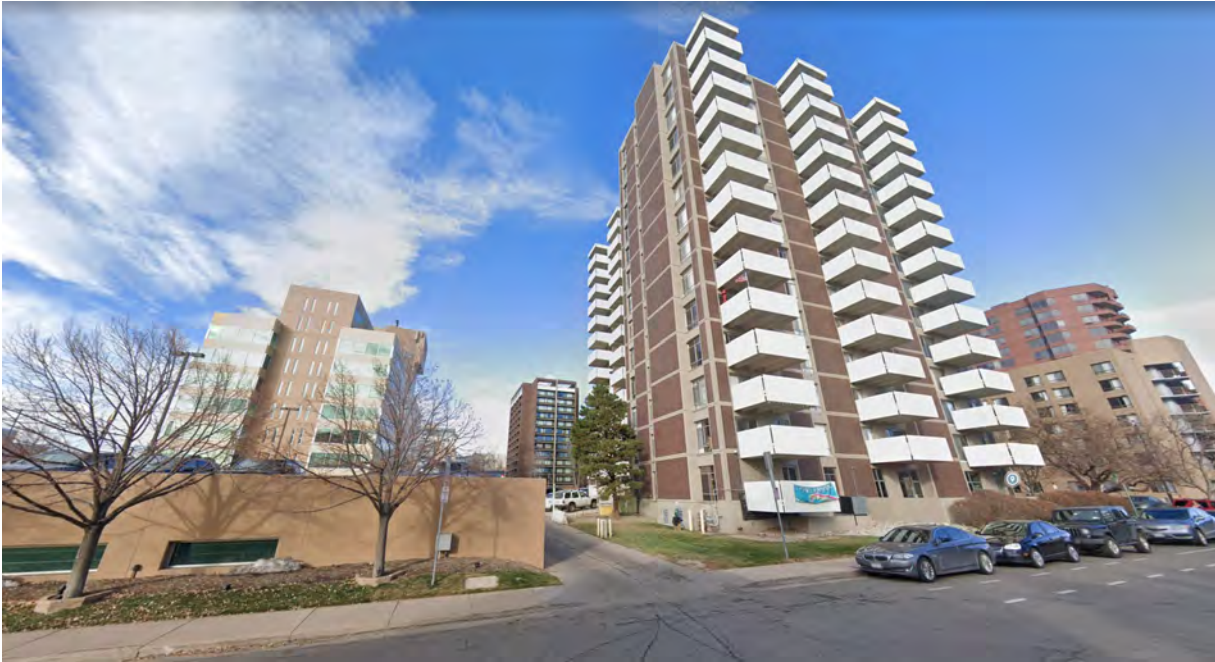
Site – from Ellsworth Avenue, facing north
