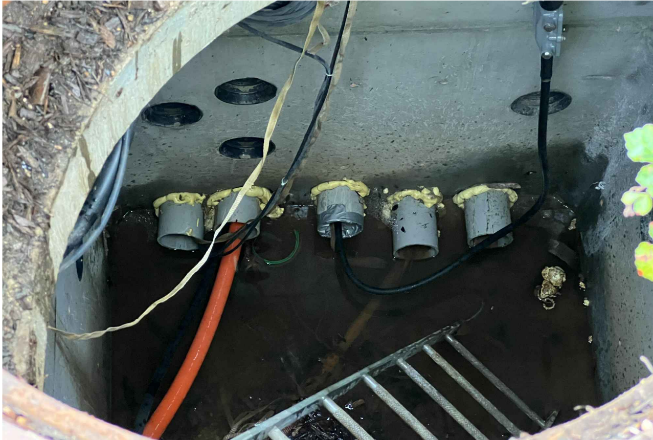
3 | CONDUIT IN COMMUNICATIONS MANHOLE
