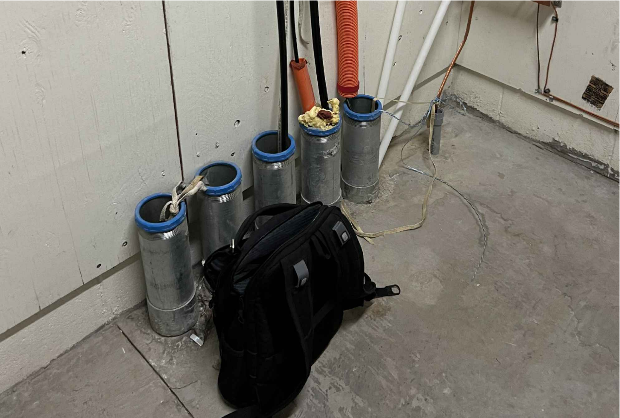
1 | CONDUIT STUB UPS IN ROOM B100
