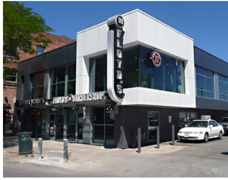
Cube Building - The Creative Farm
