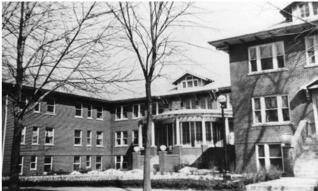
Figure 4. View of west and center projecting wings and west sunroom. c. 1924. Note pergola at raised porch, exposed brick at stairway walls and porch brick enclosure rail. Center wing entry with gable canopy at far right. SOURCE: National Register listing.
