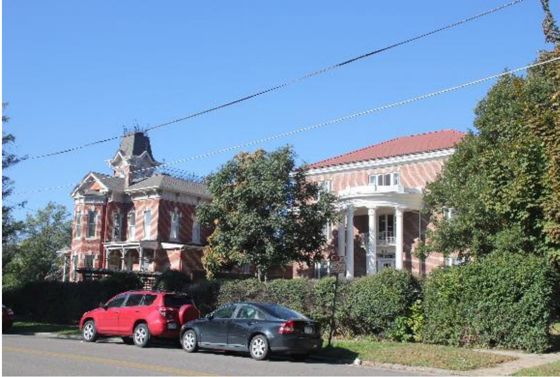
Figure 23. Bosler-Yankee House with tower restored and comprehensive rehabilitation complete. Patient Apartments at right. Photograph by Paul Cloyd, October 2018
