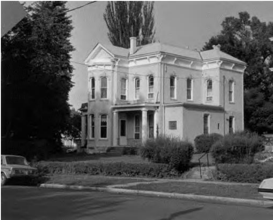
Figure 12. 1983 northeast view of the Bosler Yankee House. Brick now painted and tower is absent. SOURCE: Denver Landmark Nomination, Denver Public Library call number X-27137. Photograph by Christine Smith.
