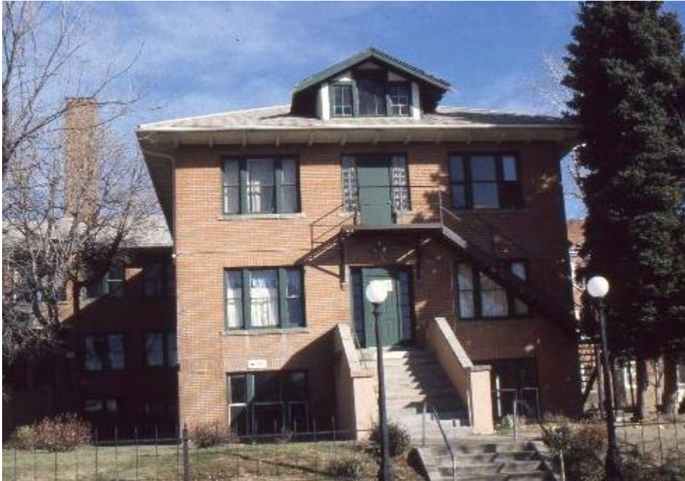
Figure 14. South facade of east wing, November, 1994. The metal fire stairs were installed in 1972. Note the second-floor doorway has been modified with adjoining glass block sidelights. SOURCE: Denver Public Library, call number 5DV2768OAHP, History Colorado, Office of Archeology and Historic Preservation. Photograph by Tom Simmons, Front Range Associates Inc.
