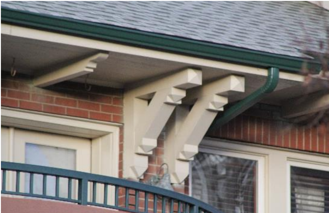
Figure 28. Detail of decorative knee brackets and joist tail bracket at eaves above west sunroom. Photograph by Paul Cloyd February 2018.
