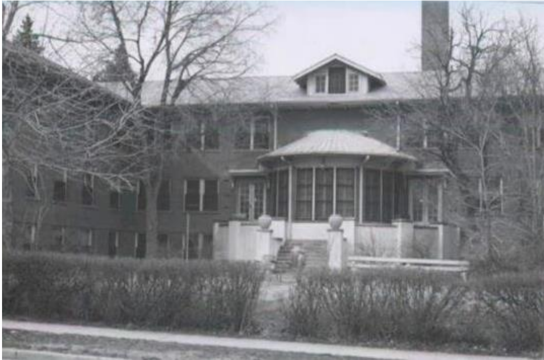
Figure 10. East sunroom, March 1977, Note standing seam metal roof over east sunroom. Multilight French doors with canopies situated to either side of sunroom bay. Stair side walls and porch enclosure rail now with stucco finish. SOURCE: History Colorado, from files for 1995 National Register listing, reference number 5DV.2768.
