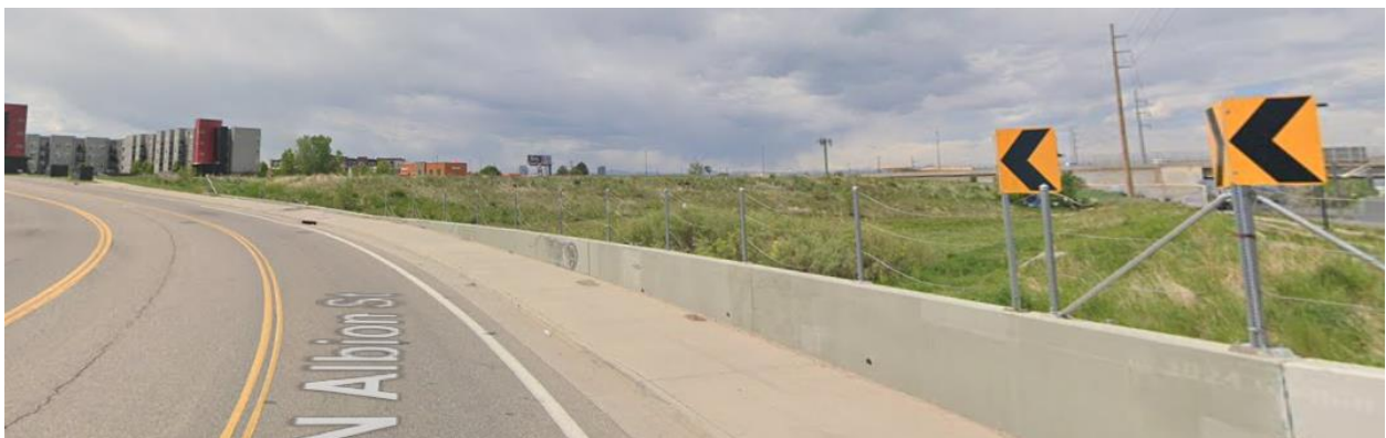
Google Image: View of the subject site looking southwest from N Albion Street.
