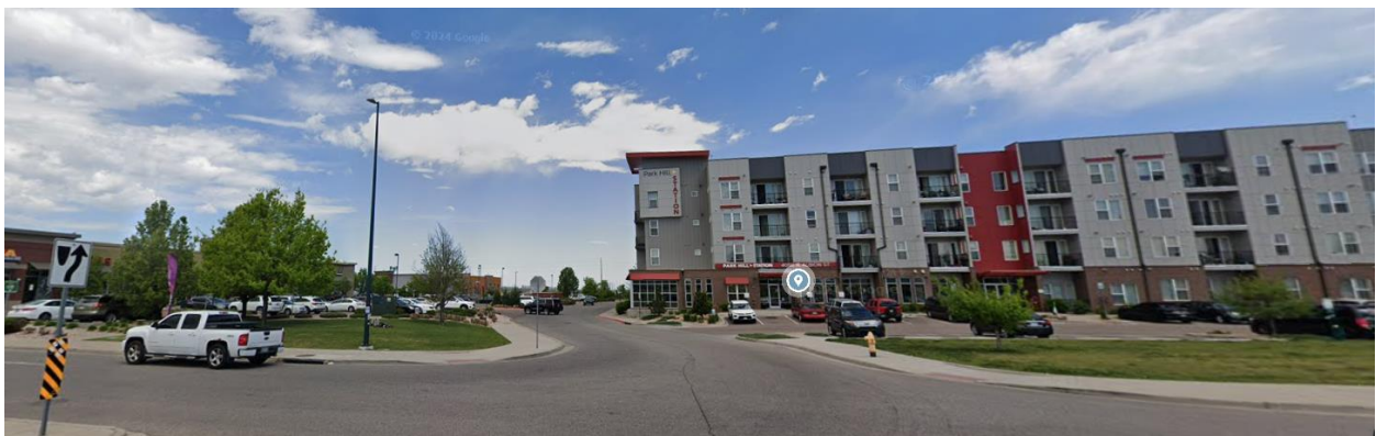
Google Image: View of the subject site looking north from 40th Avenue.
