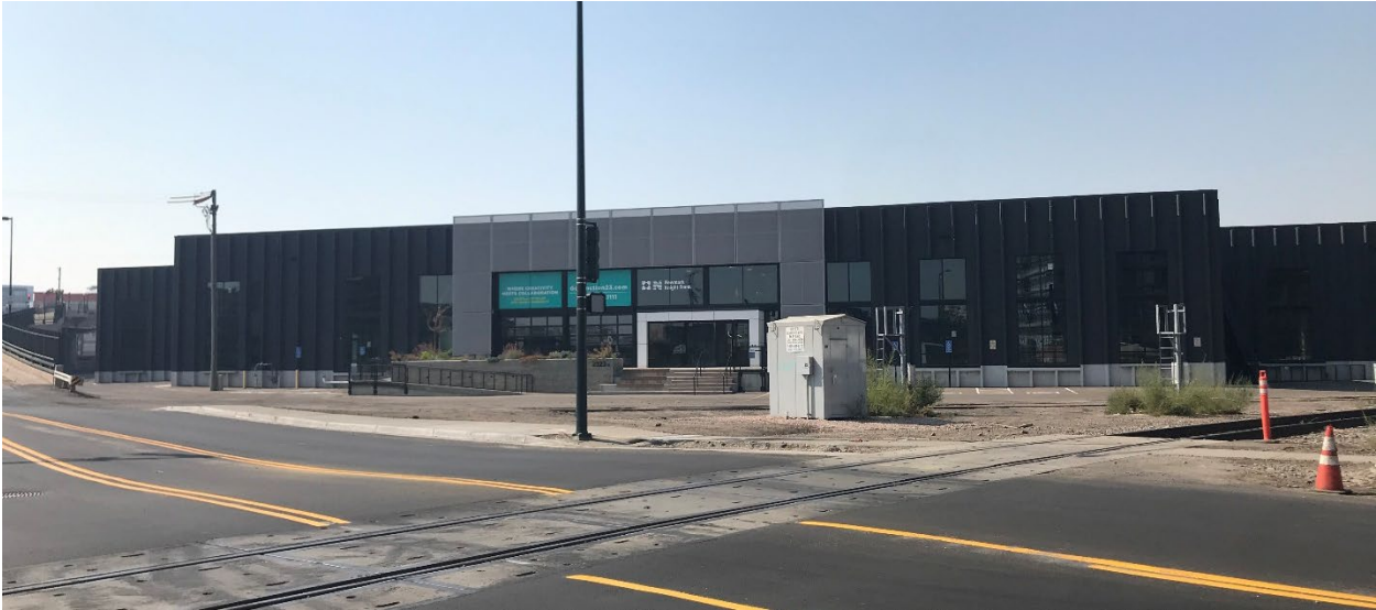
South - Looking west from Denargo Street
