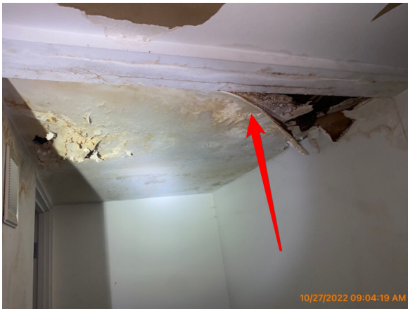
Damage with microbial growth
