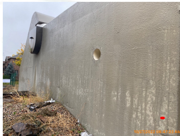
Deteriorated top coat
