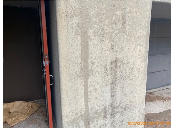
Deteriorated top coat
