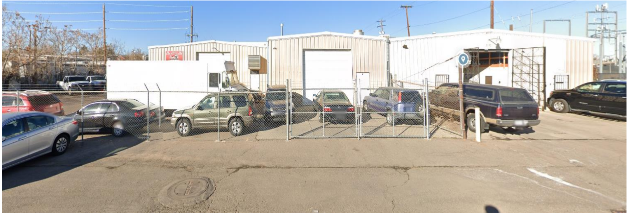
View of the subject property on North Inca Street, looking west. (Source: Google Maps)
