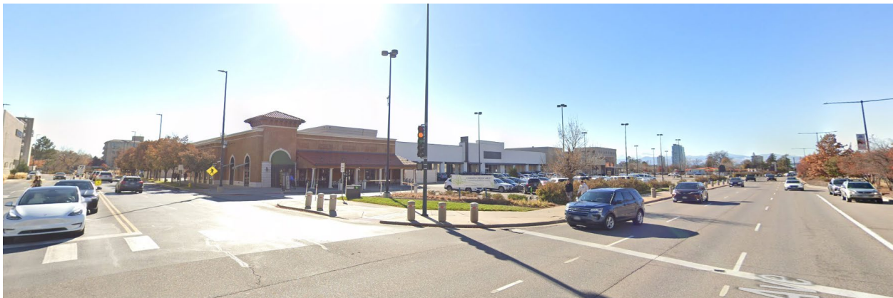
View of the subject site, looking southwest from the corner of East 1 st Avenue and Clayton Lane.
