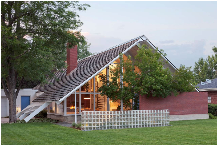
Figure 19: 618 South Monroe Way South Elevation, 2014
