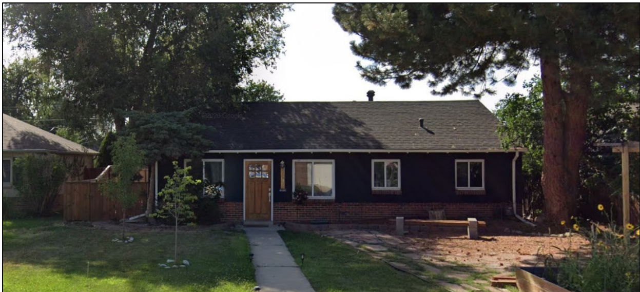
View of the subject property looking west.
