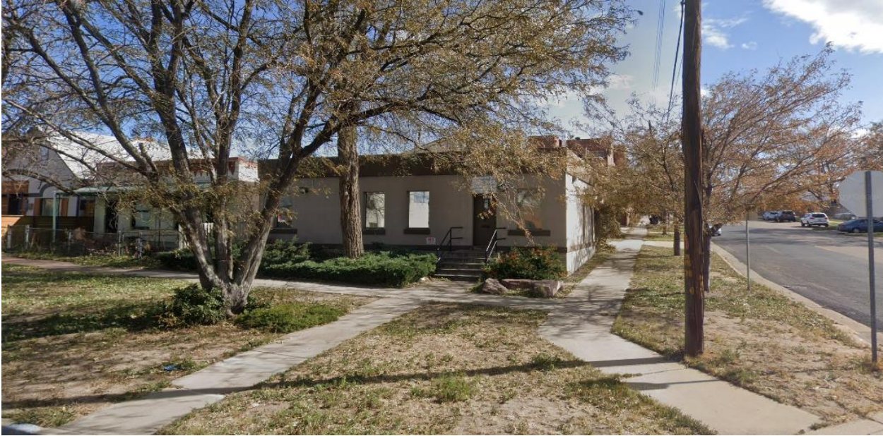
Subject property – from Mariposa Street, looking east.
