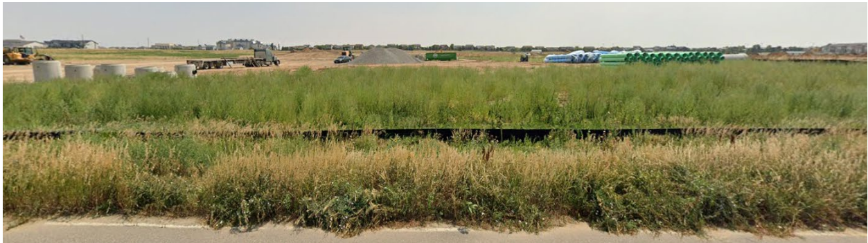
Site - Looking east from Argonne Street
