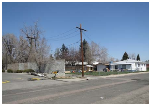
View of subject site with residential uses to the east
