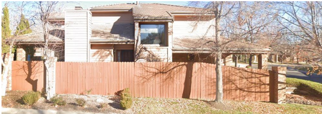
South – View of the property to the south of subject property, looking east located across East Dartmouth Avenue.
