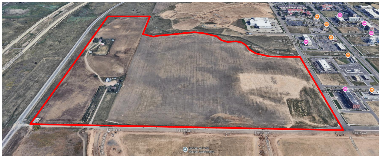
View of the property looking north.
